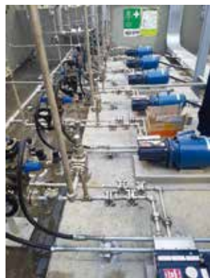
Aqueous ammonia supply pump
